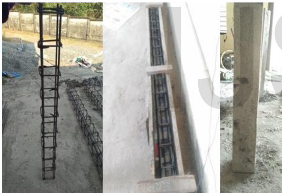
Fig 6 : Casting of short columns
