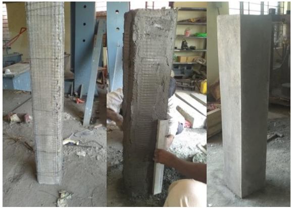
Fig 8 : Stages of retrofitting of columns
